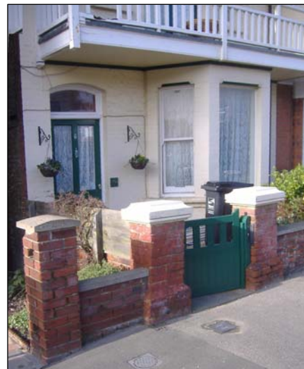
The BH boundary marker can just be seen in this photograph in front of the left-hand brick gate-pillar of number 6 Norman Road
